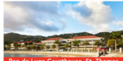
Ron de Lugo Courthouse, St. Thomas
