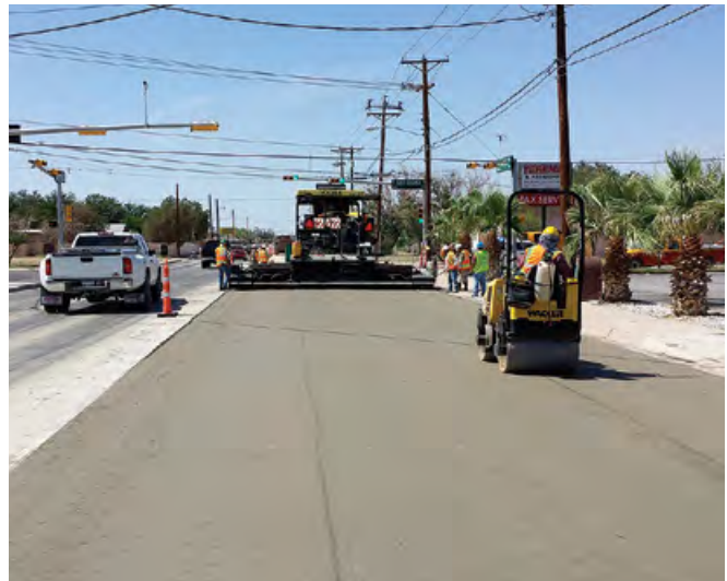
Figure 3: RCC Construction on Lamesa Drive, Midland, TX - 2014
