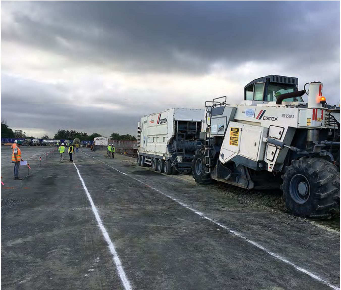
Figure 4: Full Depth Reclamation with Cement on the Crowley Terminal Facilities in Puerto Rico
