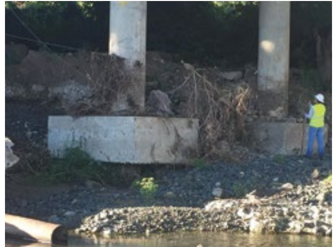
Fig. 6. Scour and exposed footing and piles at interior pier of Bridge No. 2086, Sabana Grande PR
