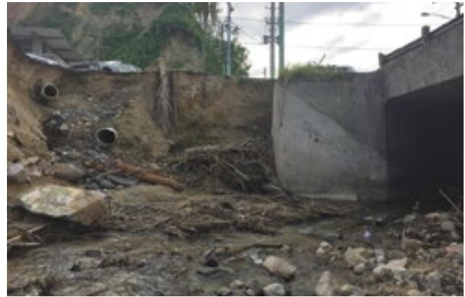
Fig. 2. Upstream embankment landslide Bridge No. 879, Utuado PR
