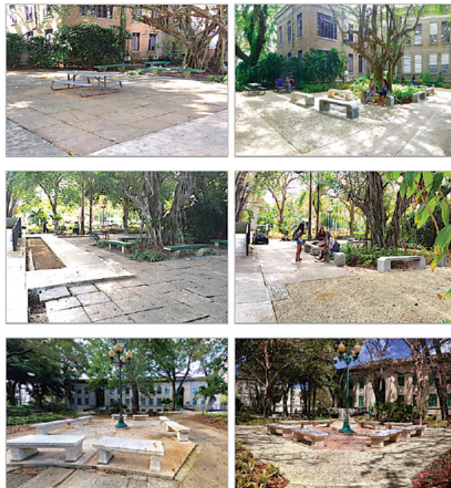
Fig. 8. Comparison views of before (left column) and after (right column) the construction of handicap accessible and environmentally friendly pervious concrete pavement on the public plaza.
