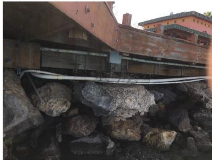
Figure 41: Exposed footing
