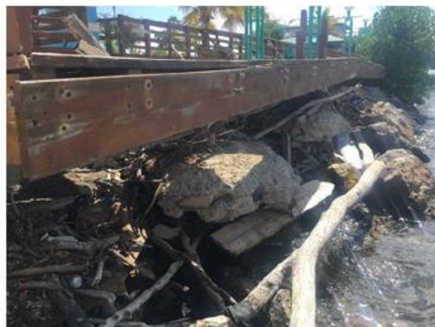
Figure 43: Damage revetment; exposed footing
