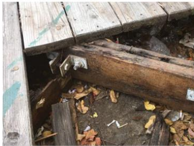
Figure 42: Damaged joist connections
